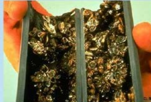
On inside of pipe
